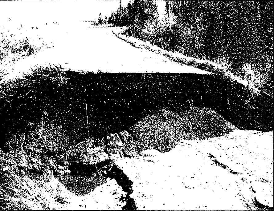
Damage caused by flooding in 2008.
